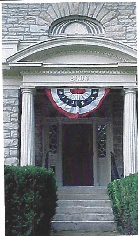
Front porch with Doric columns
