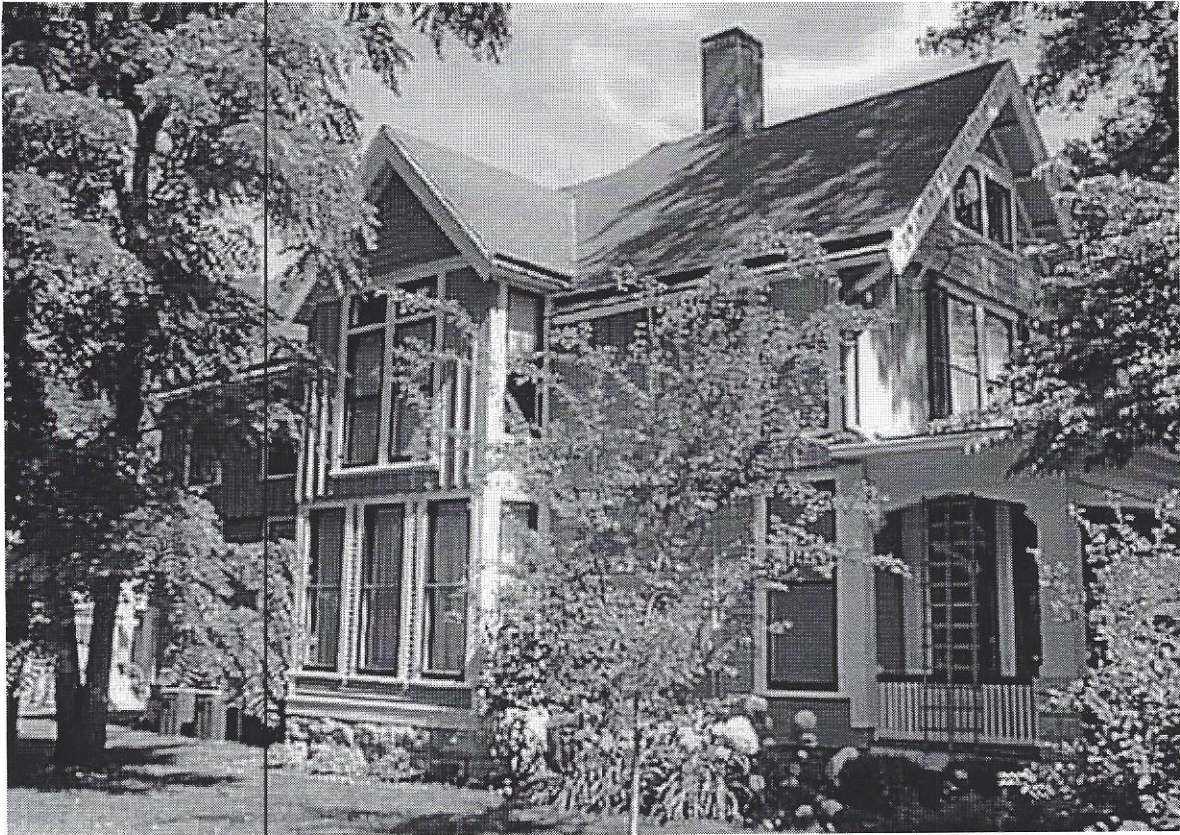
South side - projected gable and square bay, one over one double hung windows, vertical and horizontal siding, center chimney, four over four pane double hung windows on side of projected rear gable
