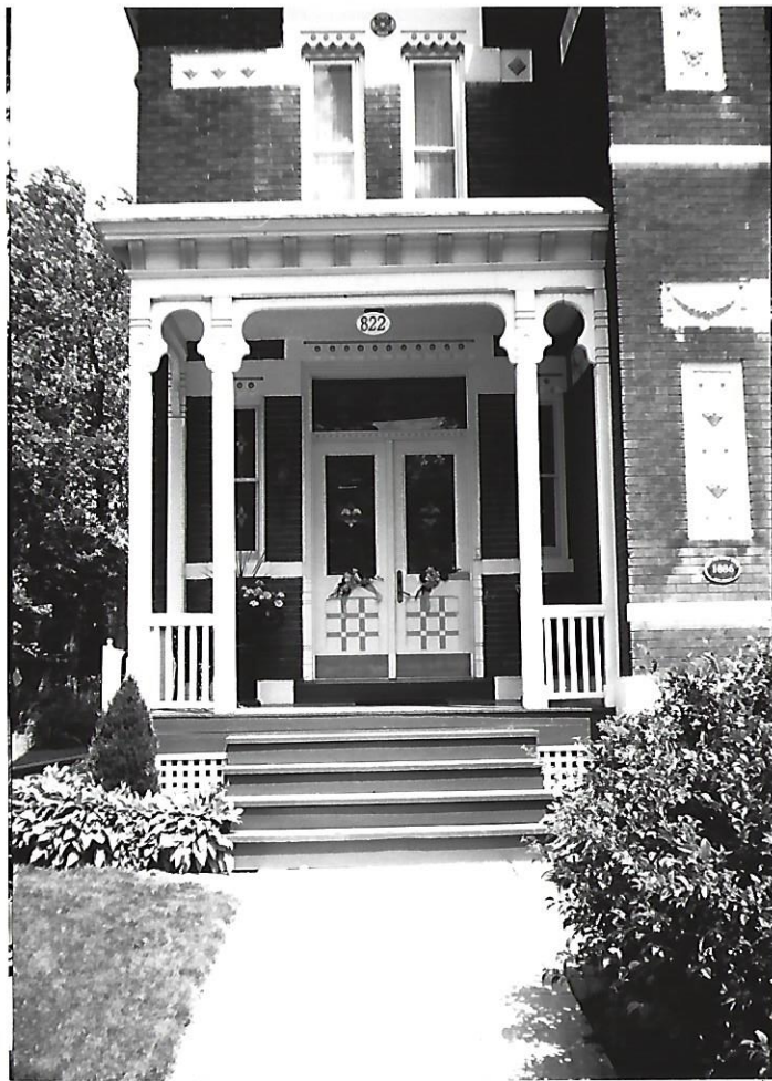
West Facade-Shows one-story entry porch with wood brackets and detailing; detail of front door opening.
