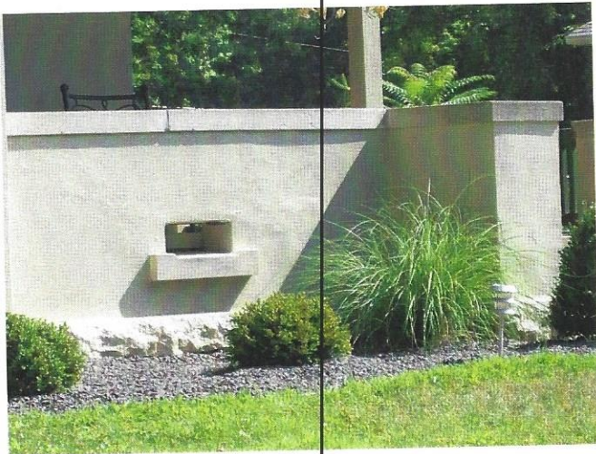
A porch detail showing a cut out design with stone sill as well as the stone cap and ashlar cut belt course that runs along the entire house.
