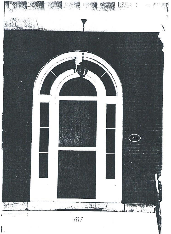
Detail of the entrance door with its semi-circular shaped opening and toplights and sidelights, the front door with a semi-circular shaped top and the stone threshold
