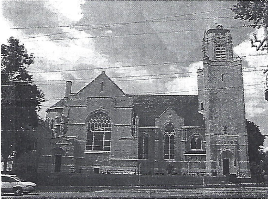
South facade - bell tower at east end, large gable with arch stained glass window, in between area divided into three sections, center one with gable top and rose window, rear entry and side of wing
