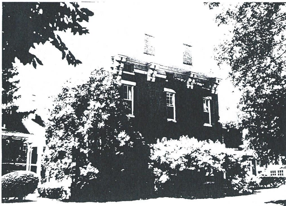
East Facade-Shows the placement of windows; two of the four chimneys; the brackets and frieze
