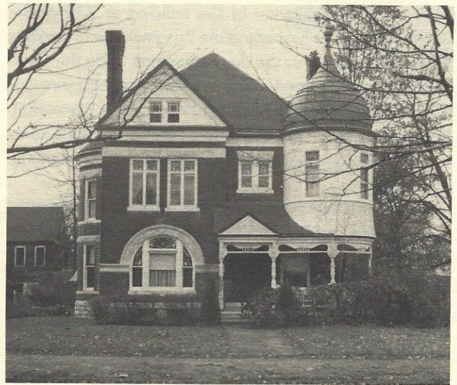
1100 State Street Architect unknown
