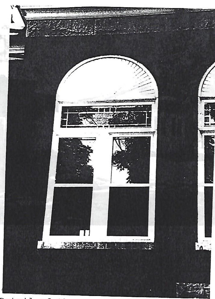
Detail of the second story window on on the West facade with the semi-circular brick arch opening, stone sill, wood sunburst carving, toplight and double sash window configuration
