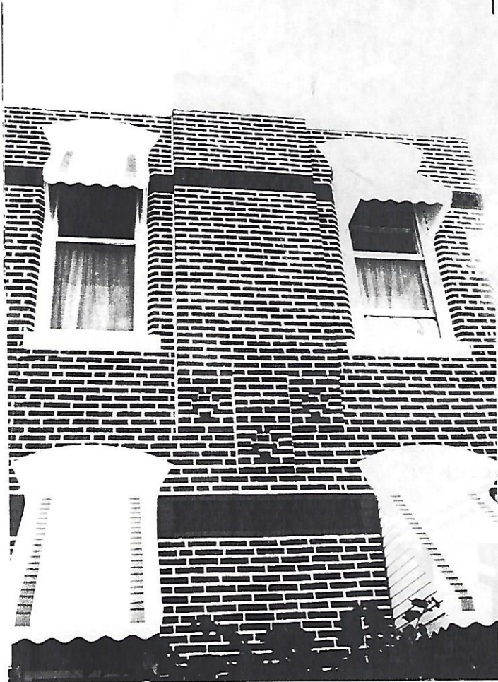
Detail of the West facade-Shows the decorative brickwork, the wood cornice with brackets and carving, the segmental brick arch windows with stone sills
