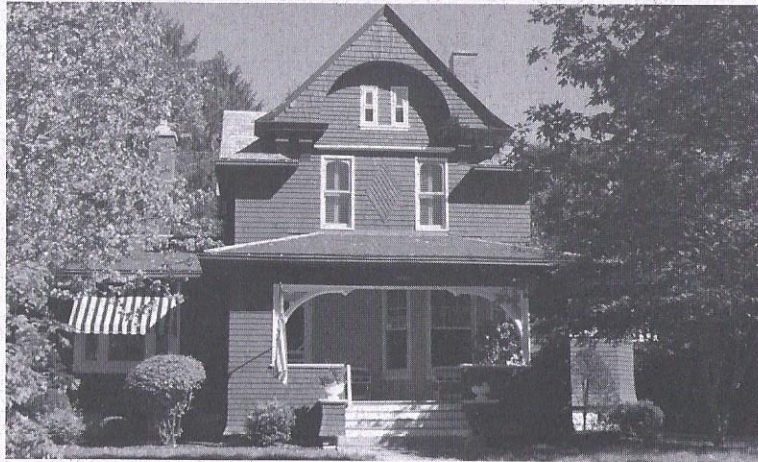
1843 Grove Queen Anne/Shingle Style • 1898 • Ernest Wood House
