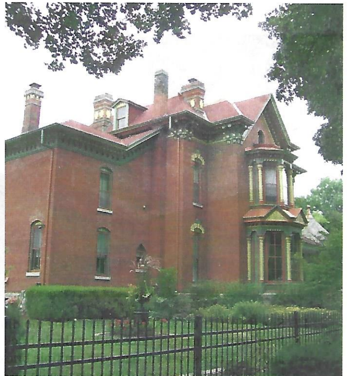
16. Addition off of east facade.
