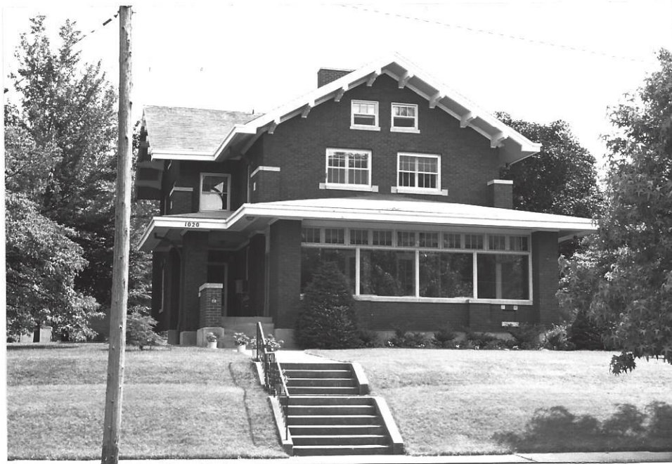
1020 Kentucky St. showing corner piers with stone caps, exposed rafter tails under wide eaves, and porch support piers
