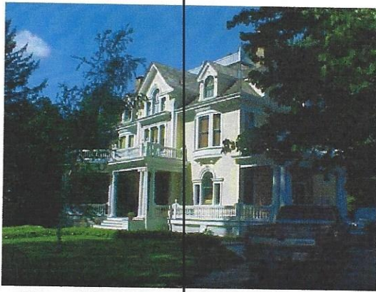
View of front façade facing East Avenue
