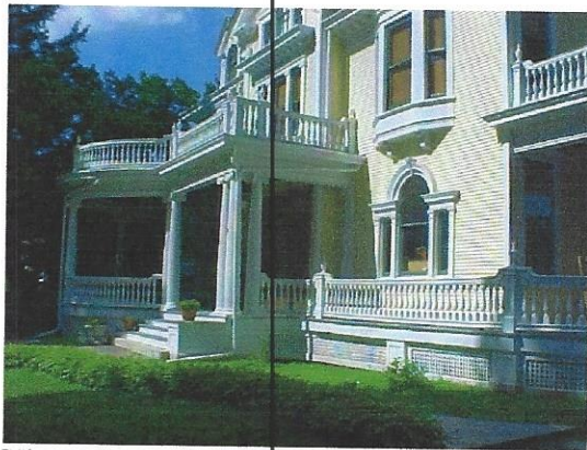
View of circular verandah and connecting promenade
