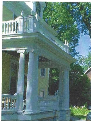
Portico with triple Ionic columns
