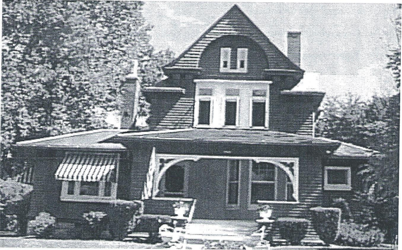
South (primary) facade - original home visible behind porch and side additions, gable with circular detail and paired windows, set of three windows on second floor
