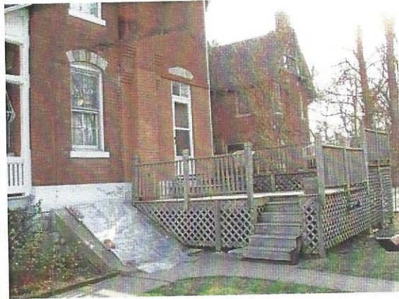
Location of proposed porch (demolish existing deck), note location of previous structure
