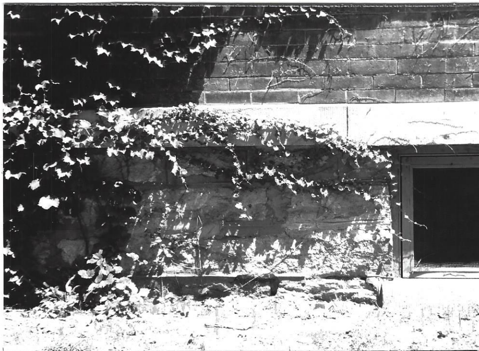
Detail of the limestone foundation, the smooth-cut stone water table, and the brick exterior wall
