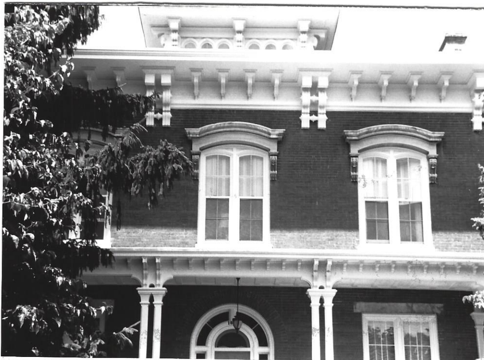
Detail of the windows on the second storey of the South facade with the stone segmental crown supported by stone brackets, and the double windows with four-over-four window panes, and stone sills
