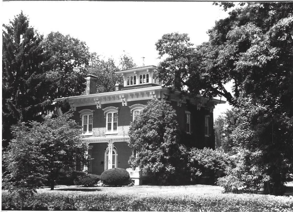
South Facade-Shows the two-story massing with a low-pitched roof; placement of the cupola and porch; the four brick chimneys on the main mass of the house
