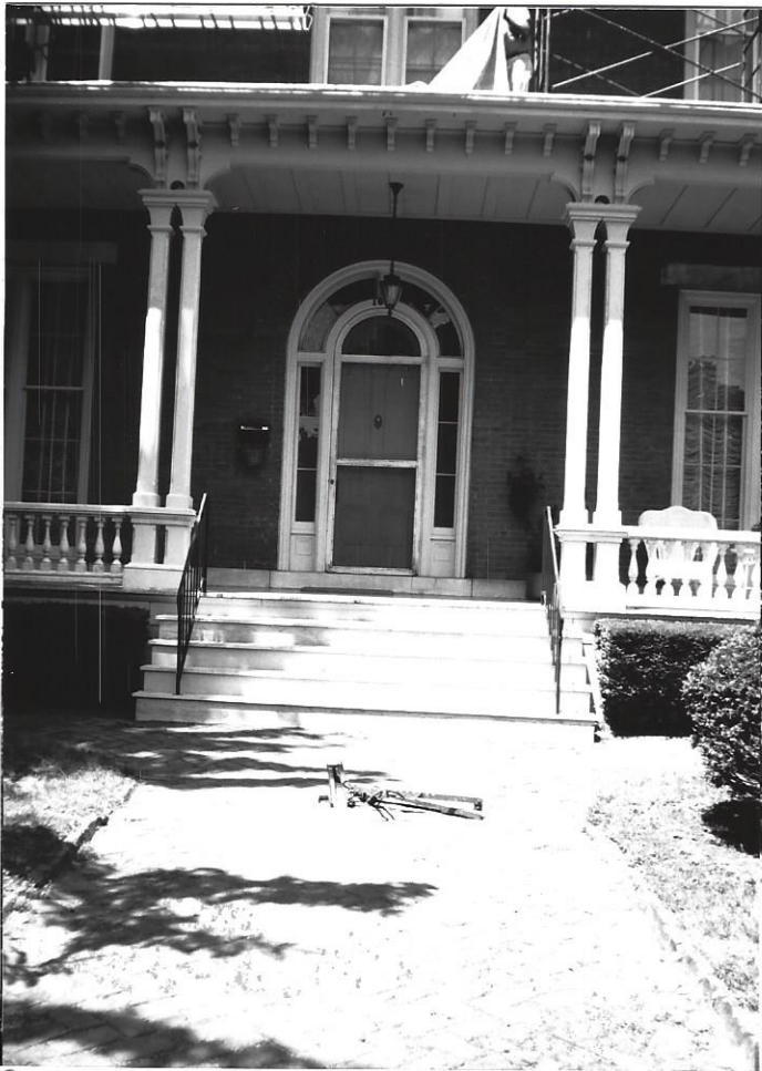
Detail showing the stone steps to the front porch, the placement of the front door, and the brick sidewalk that extends from the city sidewalk to the porch, and the stone threshold
