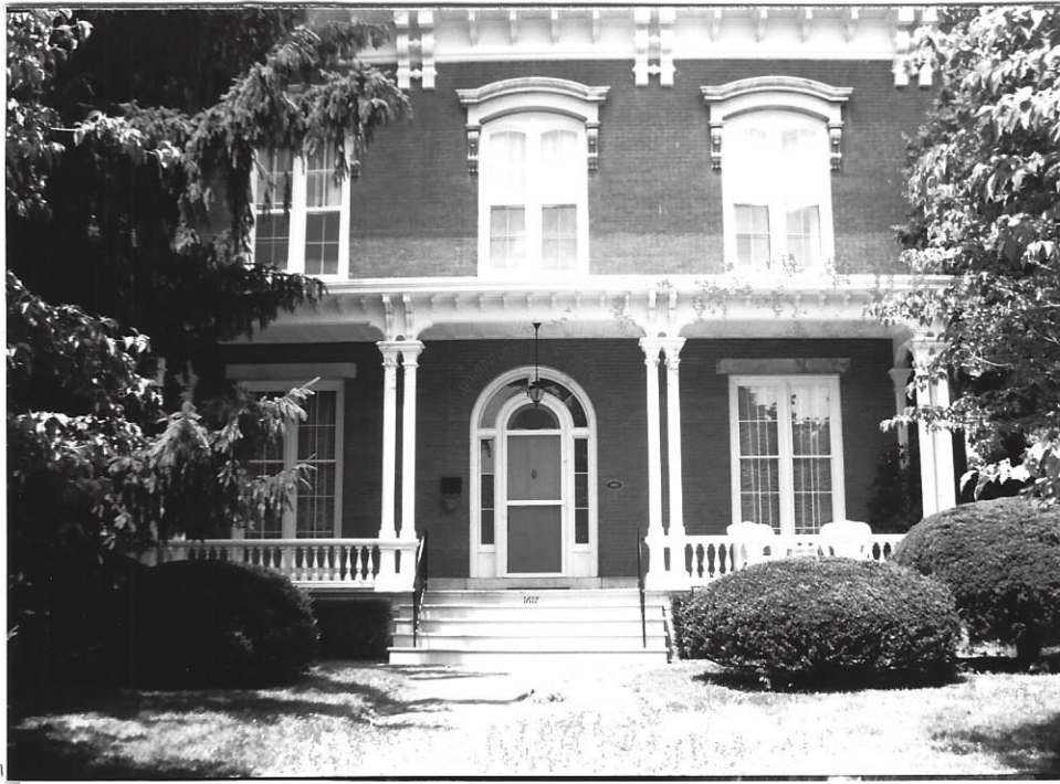
South facade-Shows the one storey full-facade porch, with its double posts, turned wood balustrade, wood rail, stone steps and brackets under the porch roof-line; also shows the placement of the front door on the facade
