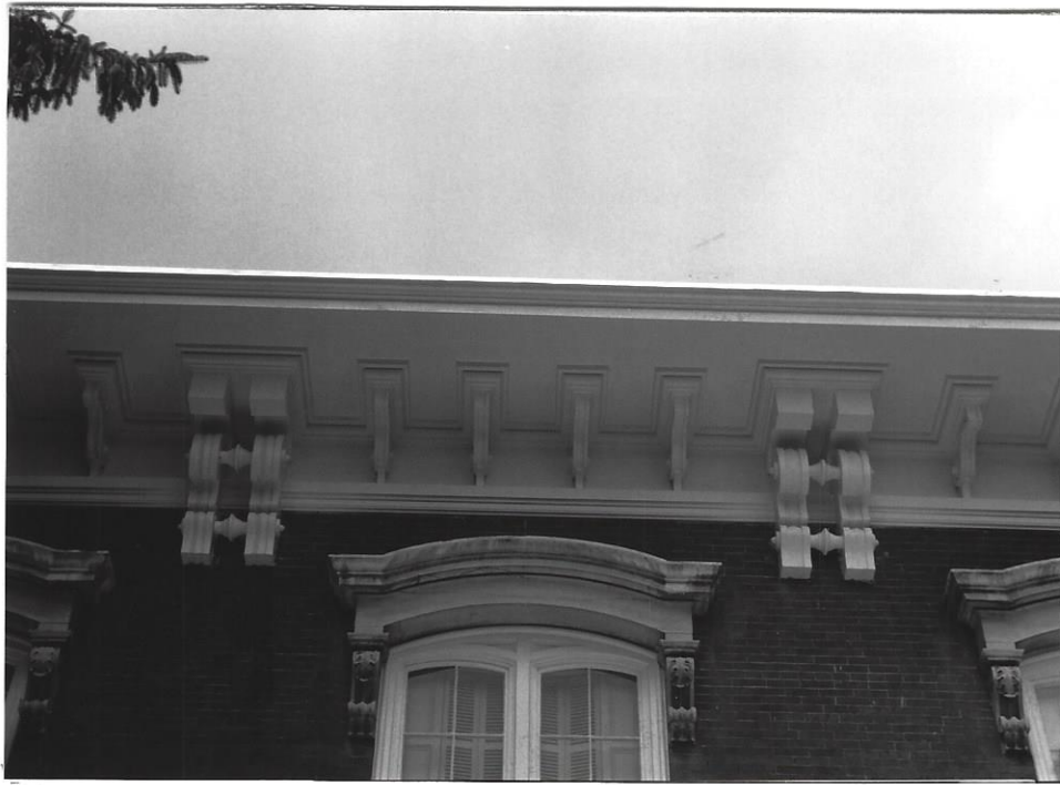
Detail of the brackets of the South facade; also shows the stone segmental window crown supported by stone brackets
