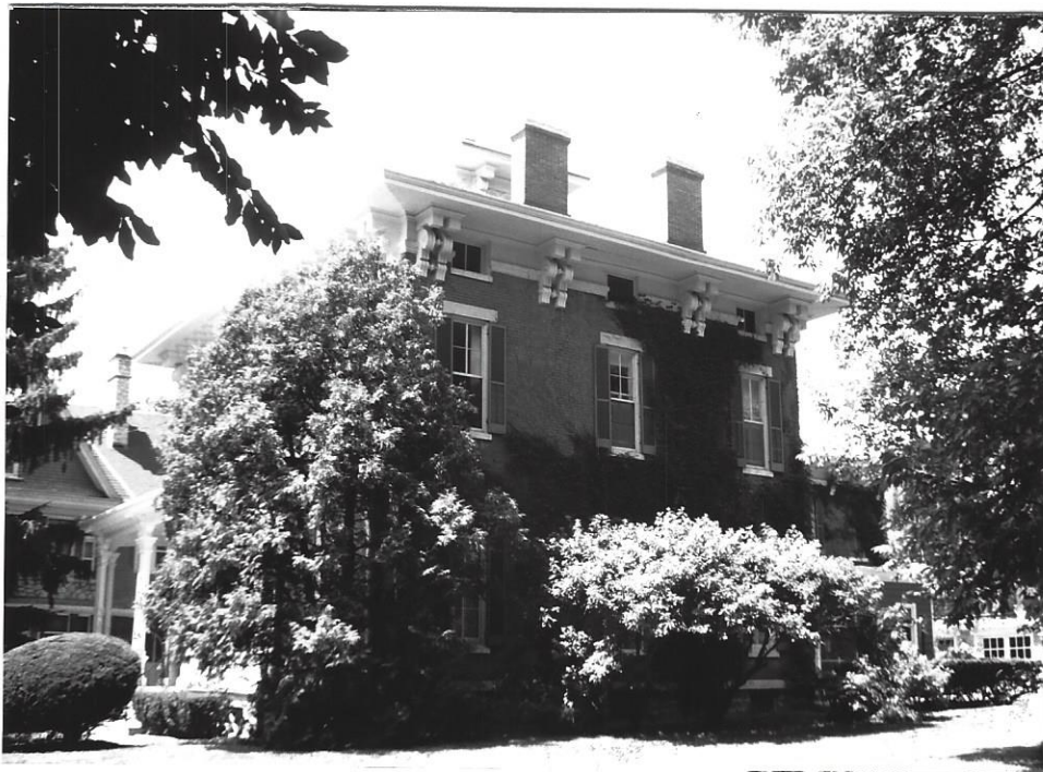
East Facade-Shows the placement of windows; two of the four chimneys; the brackets and frieze
