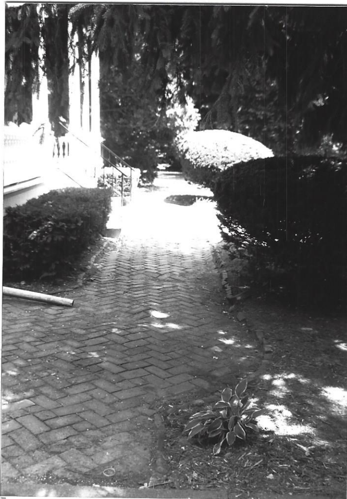
Detail of the brick sidewalk that extends across the front porch
