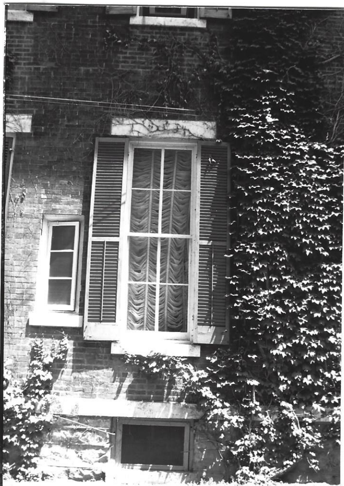
Detail of typical window found on the East, North, and West facades with stone lintel and sill, and four-over-four window panes
