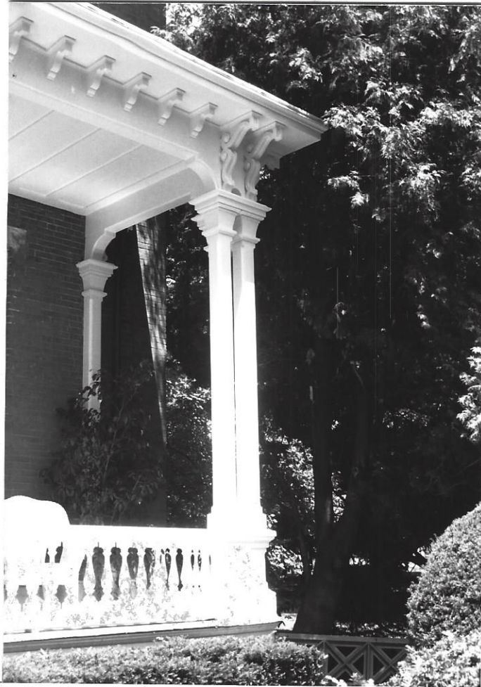
Detail of the double posts of the porch as well as the turned wood balustrade, the wood rail, the brackets, and the single engaged post supporting the porch roof at the brick wall surface
