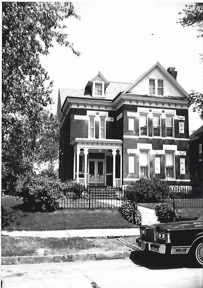
West Facade-Shows massing; primary hip and secondary gable roof; window configuration; dormer placement; one-story entry porch placement.
