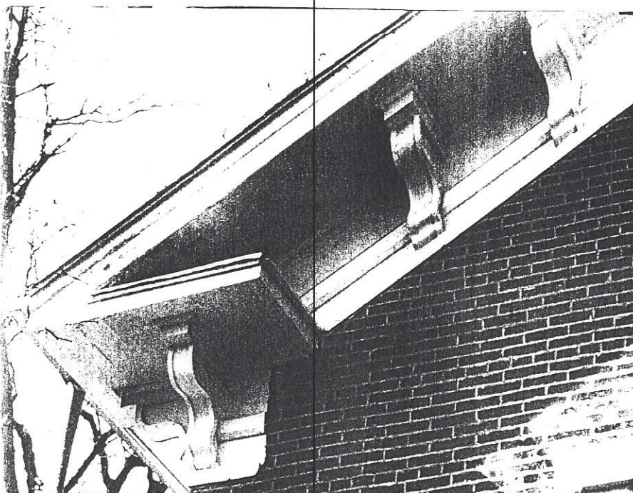
Raking cornice with brackets at the east and west gables.
