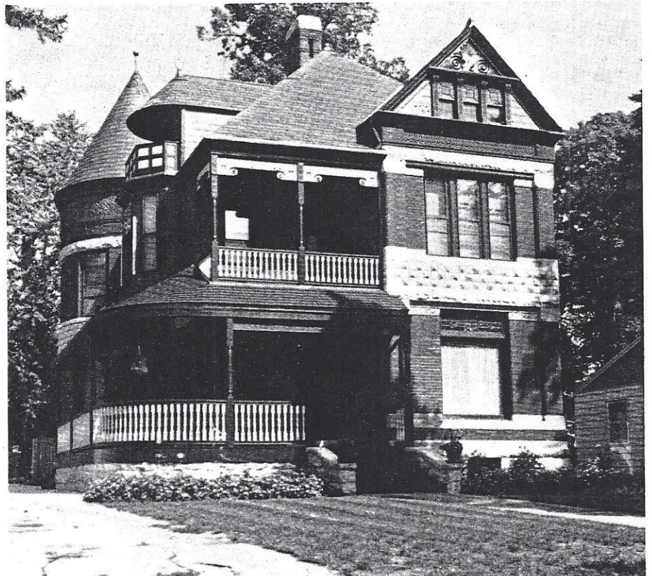
The reconstructed porch and historic paint scheme revived the century-old Musselman house. Because the restoration was completed under federal guidelines, the owner qualified for a twenty percent income tax credit.
