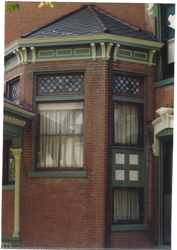
Above: East bay window. Note bottled glass windows in upper lights and slate roof.
