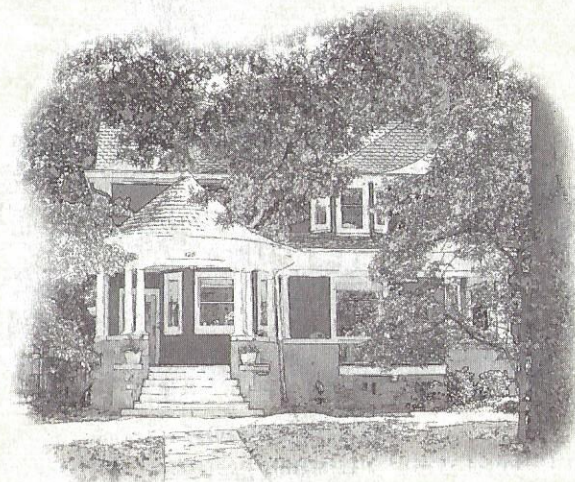
125 East Avenue Queen Anne Style • 1897 Architect: Ernest M. Wood James and Florence Neilson House
