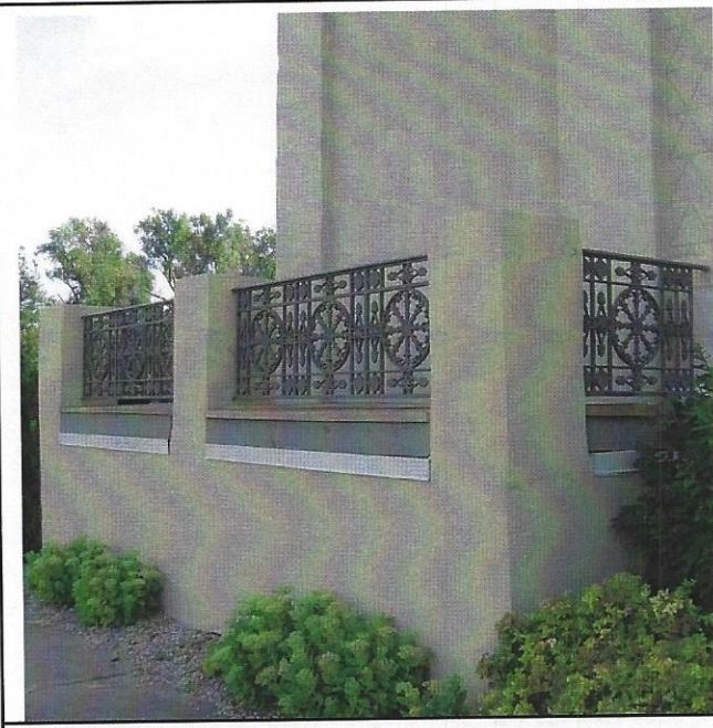
26. Porch on northwest with stucco piers and decorative iron balustrades.
