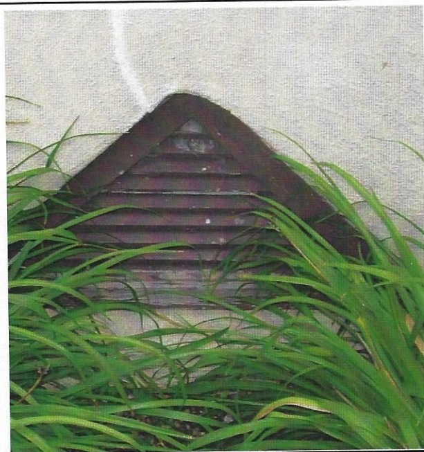
28. Wooden louvered vents at foundation level.
