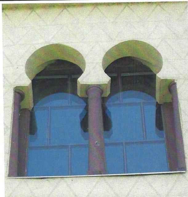
27. Double horseshoe arch with center wooden column and flanked by two engaged wooden columns on second level of the west façade.
