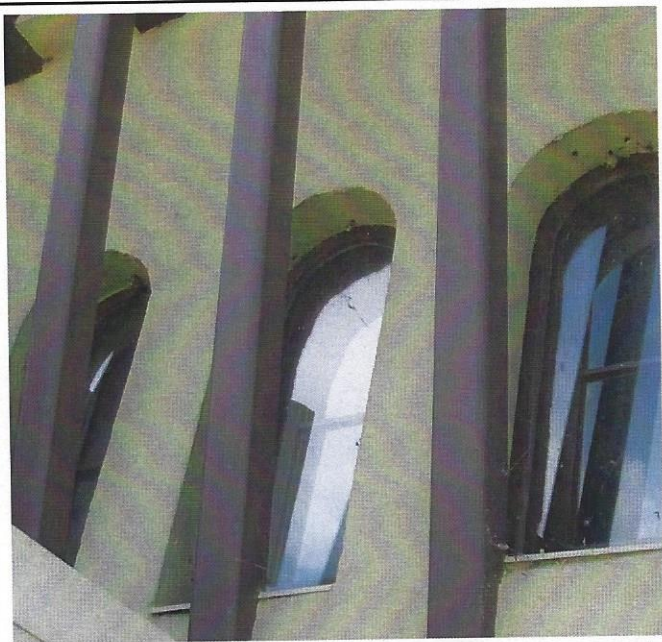
9. Three rounded arch windows behind wooden support brackets on the north façade.
