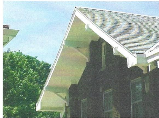
South regular pitch craftsman gable with recessed panel fascia boards.
