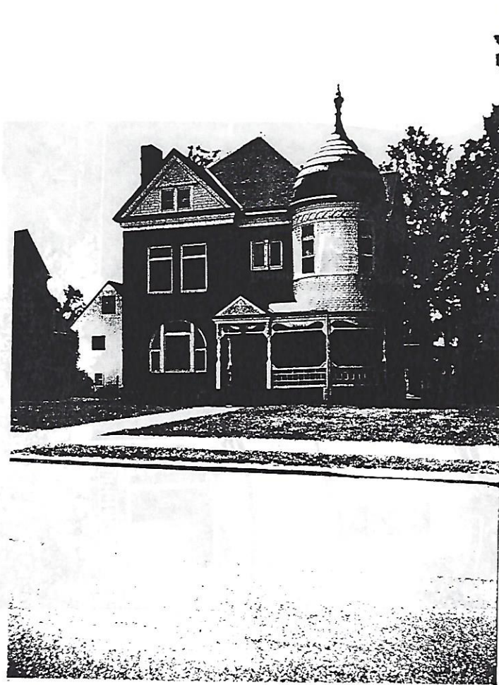
North Facade-Shows massing; primary hip roof with secondary gables; tower with dome and finial; wrap-around porch; window configuration; materials
