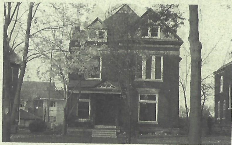
1217 Park Place Queen Anne Style • 1890 Henry & Augusta Pfeiffer House Architect: John Batschy
