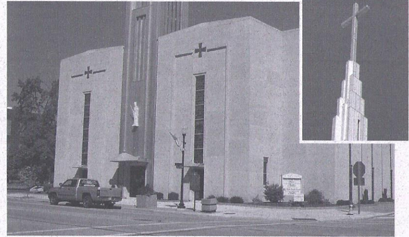
117 N. 7th St. Boniface Church Mid-Century Modern • John Benya, Architect
