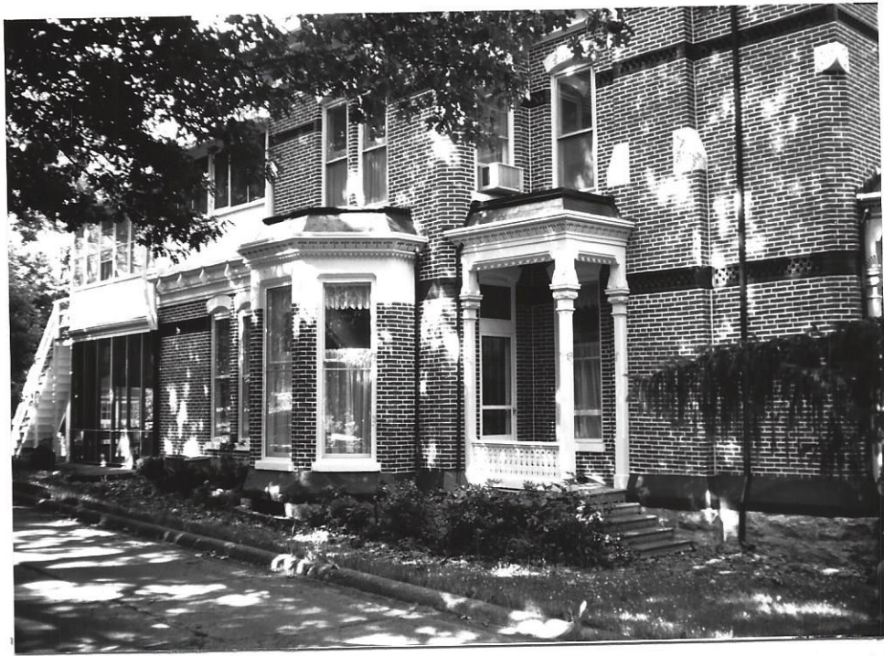
Detail of the East facade-Shows the entry porch with wood posts, rail, balustrade and carving; also shows the one story bay with its wood carving, and windows with stone sills and lintels; also shows decorative brick beltcourses
