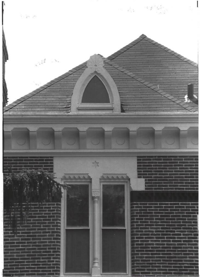
Detail of the North facade-Shows the Lancet-shaped dormer with shell carving at the peak, the wood cornice, brackets and carving, and the second floor window with stone sill, and lintel and carving
