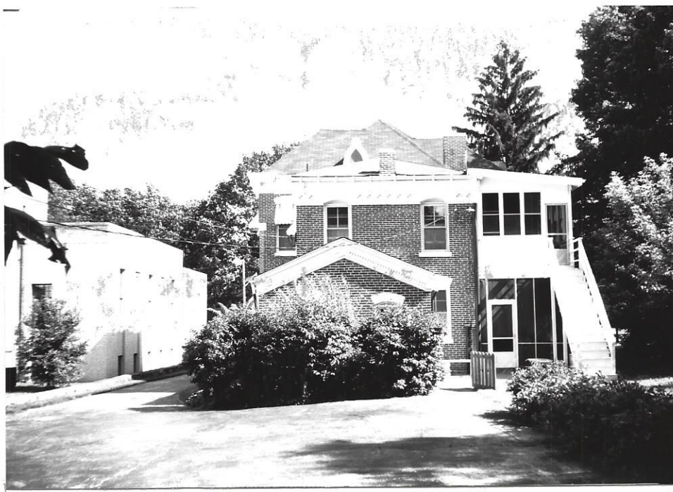
South facade-Shows the two story brick wing and the one story brick wing on the two story wing, placement of the chimneys, window openings and the lancet-shaped dormer
