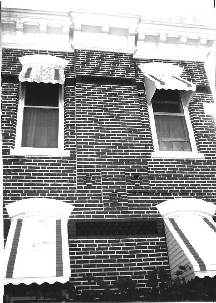
Detail of the West facade-Shows the decorative brickwork, the wood cornice with brackets and carving, the segmental brick arch windows with stone sills
