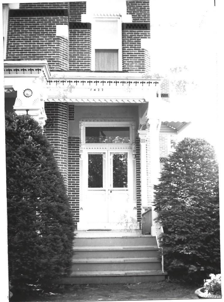
Detail of the North facade-Shows the front double doors with scalloped header, full toplight, stone threshold, and all carving on the wood framework; also shows the wood steps and platform of the porch and the carving on the porch
