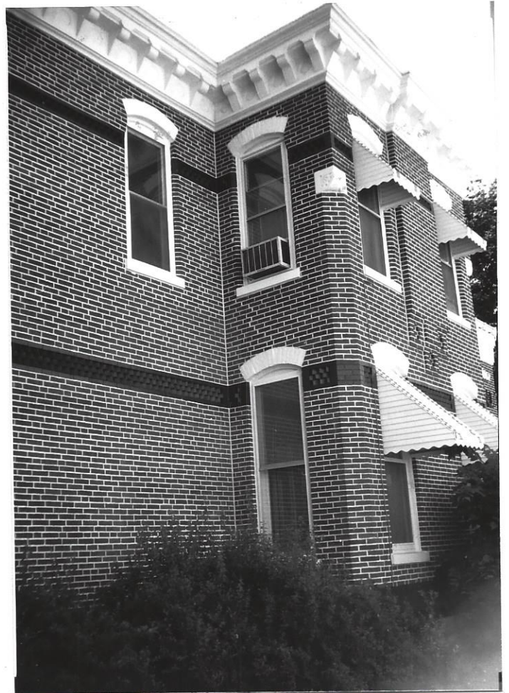
Detail of the West facade with wood cornice, brackets and carvings at the roofline, the decorative brick belt-courses, and segmental brick arch windows with stone sills
