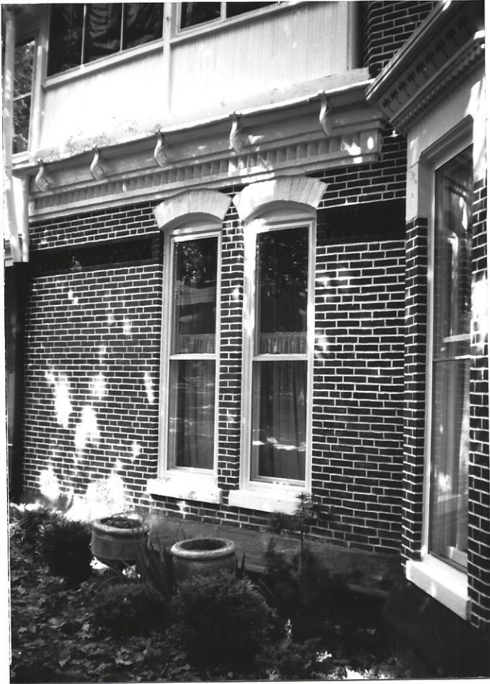
Detail of the East facade-Shows the decorative wood cornice, the decorative brick beltcourse, the segmental brick arch windows with stone sills
