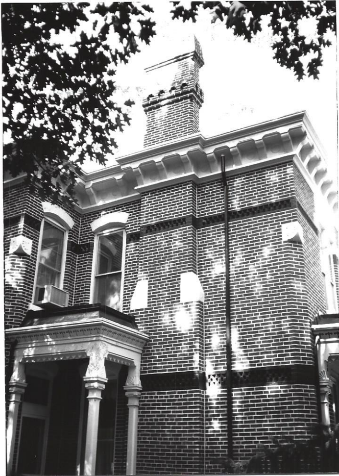
Detail of the chimney on the East facade with decorative brick and stonework
