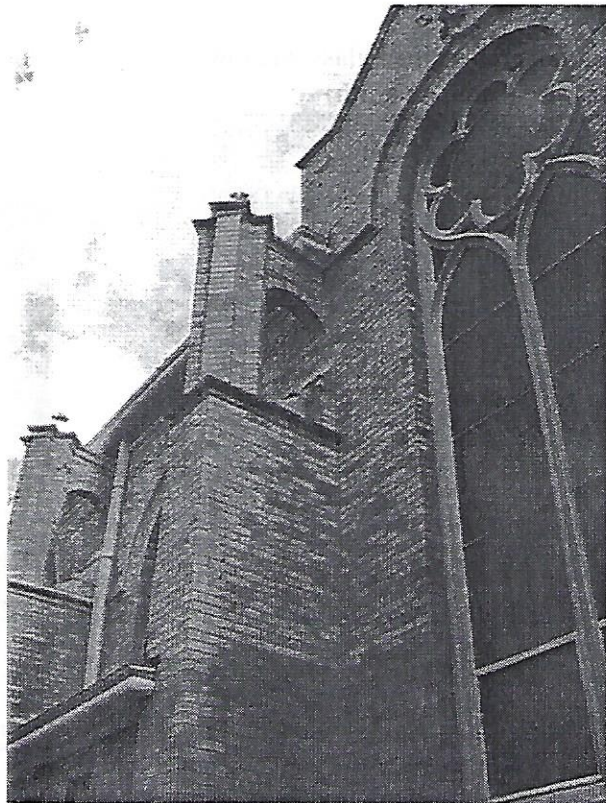
in between section divided into three sections - (south side, north is mirror) - arch stained glass windows, rose window in center, stone detail, stone water table
