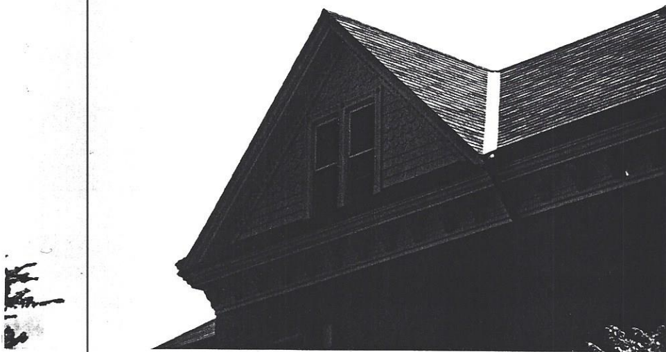
Detail of the North facade gable with wood shingles & decorative wood carving
