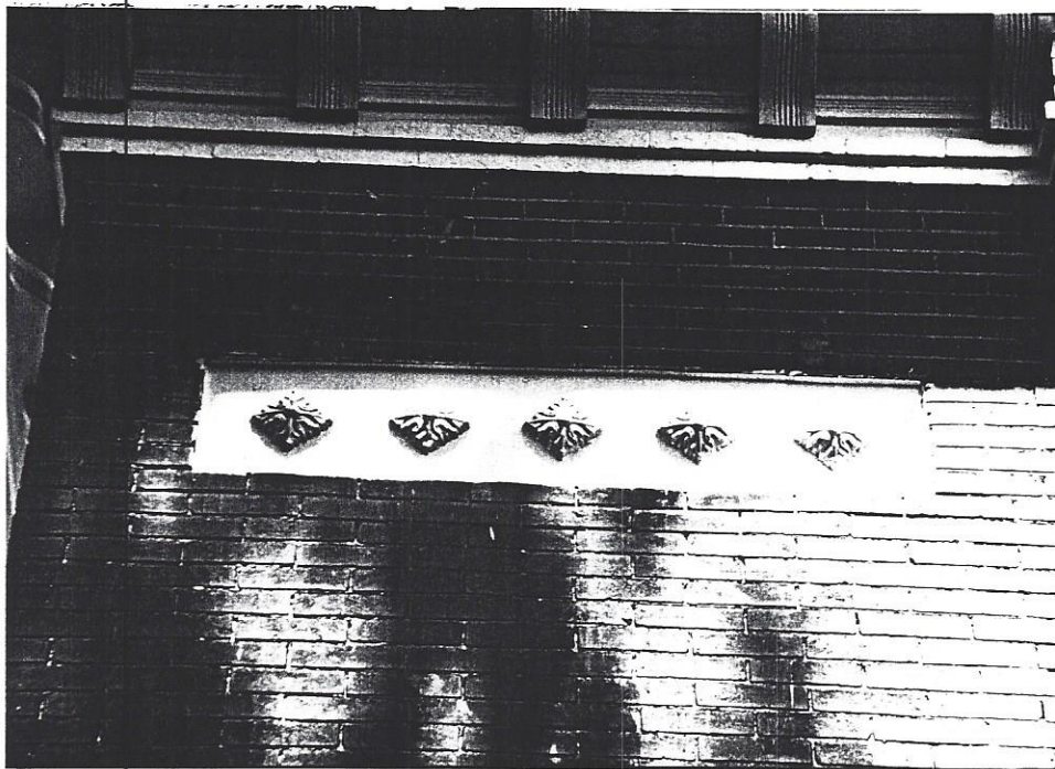
Detail of the stone banding on the South facade with 5 carved decorations. There is a matching band just below on the first story
