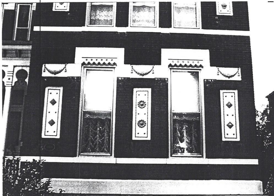
West Facade-Shows window detail with stone beltcourses; stone and pressed metal insets; smooth-cut stone watertable.
