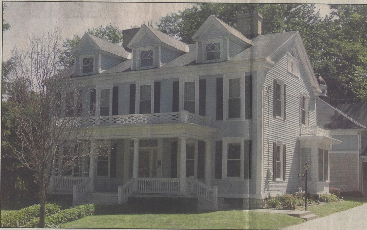
The Mena family home at 120 N. 18th in Quincy is a classic example of Federal style architecture. It features Doric columns on the porch, three dormers with dentil molding below the cornice and shuttered windows throughout. H-W Photos/Mike Badamo
