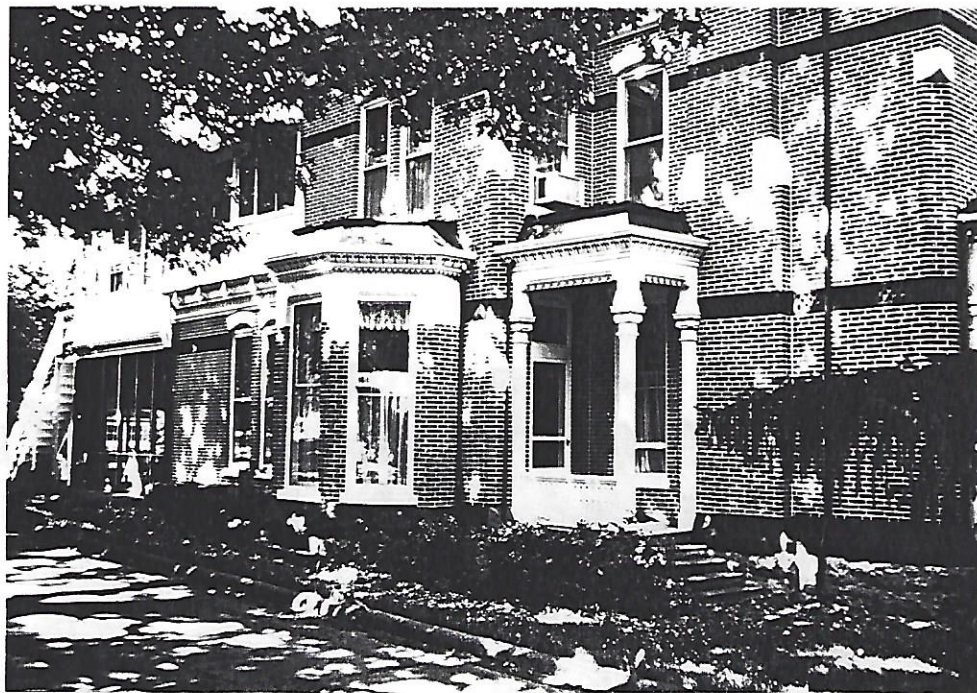
Detail of the East facade-Shows the entry porch with wood posts, rail, balustrade and carving; also shows the one story bay with its wood carving, and windows with stone sills and lintels; also shows decorative brick beltcourses
