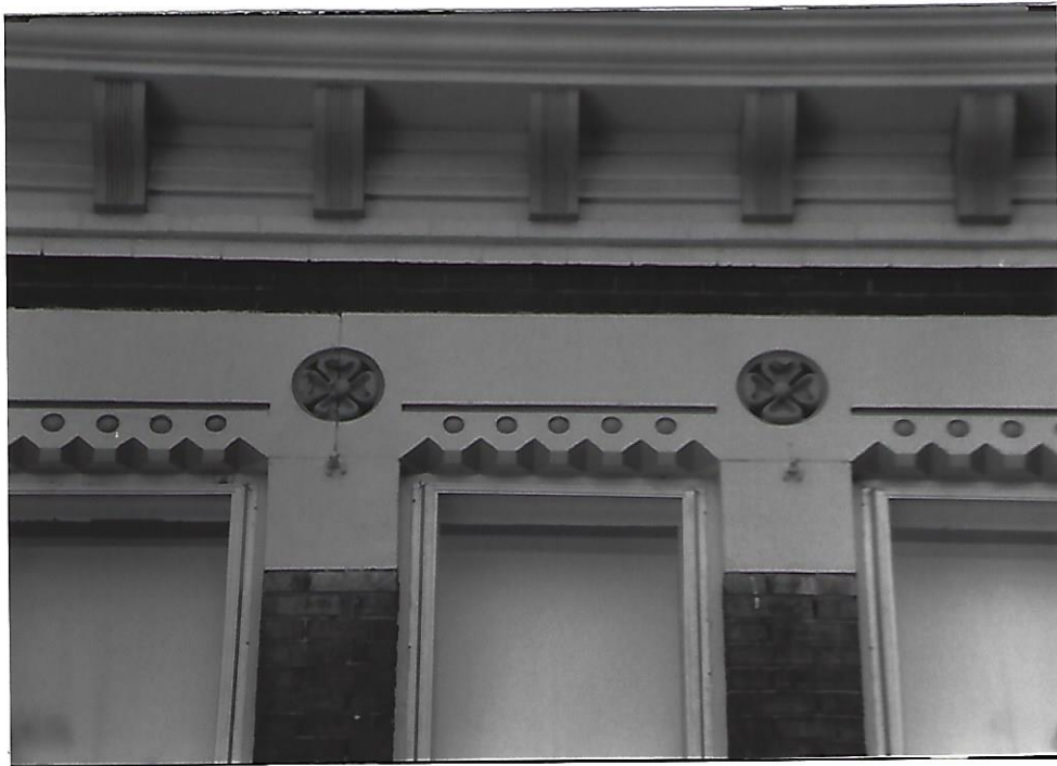
Detail of the second story window headers on the West facade—Shows the rosettes, scalloping and bead carvings in the stone; also shows the carved wood brackets at the roofline
