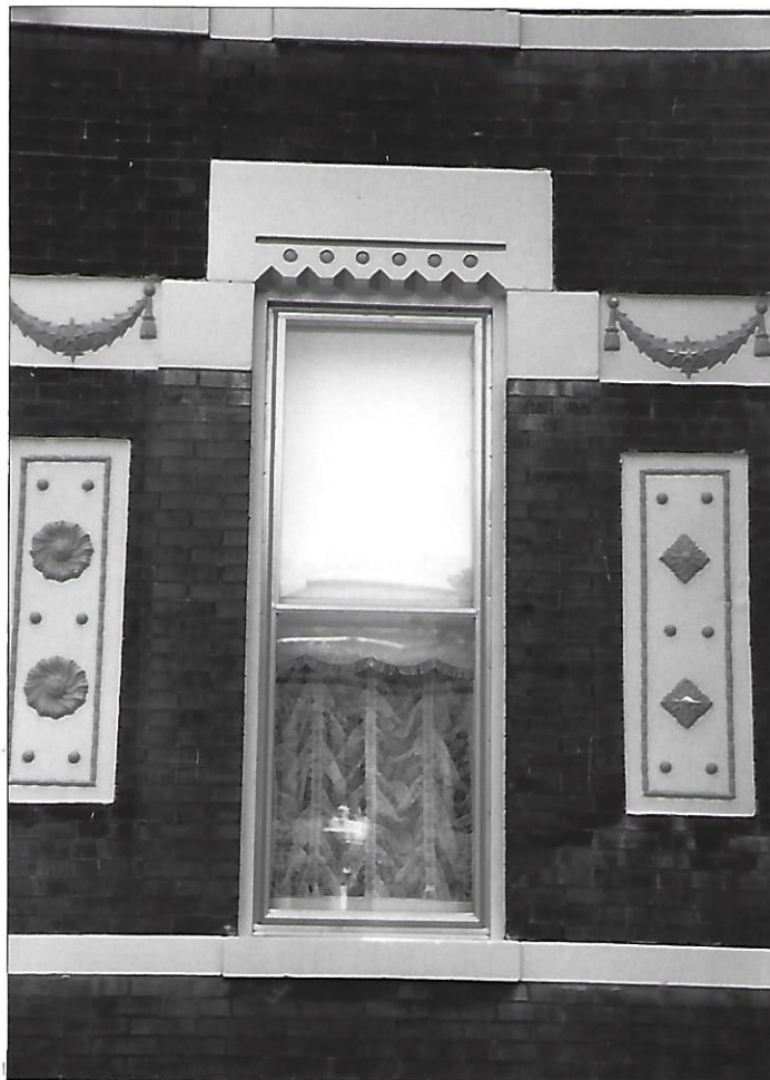
Detail of first story window on the West facade—Shows the scalloping, beading, swags, and other carvings in the stone headers and bands; also shows pressed metal panels
