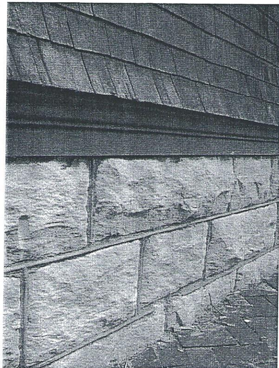
foundation with molded mortar
