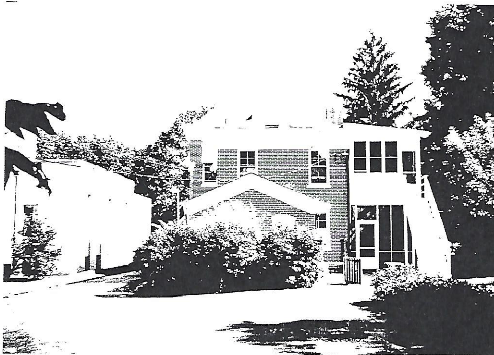
South facade-Shows the two story brick wing and the one story brick wing on the two story wing, placement of the chimneys, window openings and the lancet-shaped dormer
