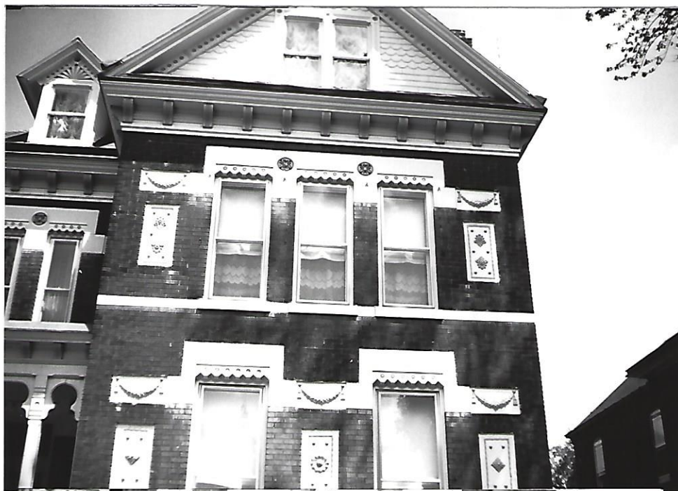
West Facade-Shows window detail with stone beltcourses; inset stone and pressed metal panels.
