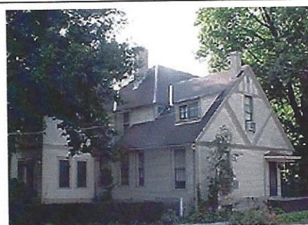
Northwest corner, stone foundation, decorative half timbering
