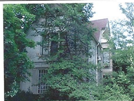
Southeast (front) side
