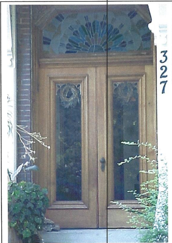
Fanlight over front double doors
