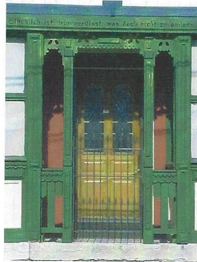
Front entrance with original iron gate from first St. Boniface Church.
