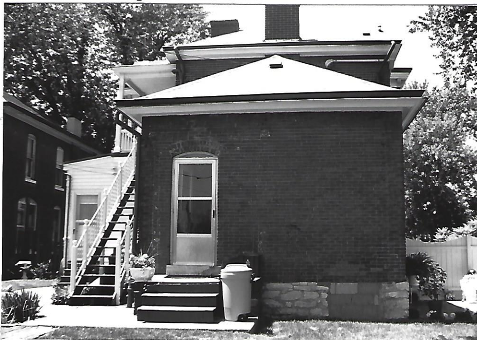
East Facade-Shows the one-story brick addition on the rear
