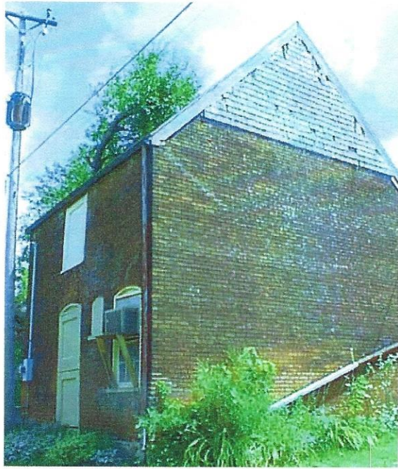
Carriage house - alley entry, brick relieving arch lintels
