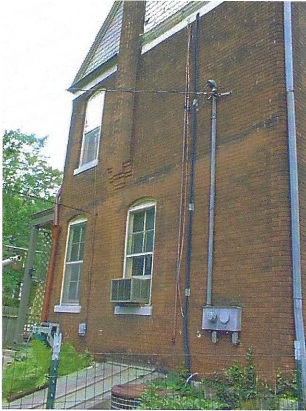
North side - chimney detail, four over four sash windows, flat segmented arch lintels
