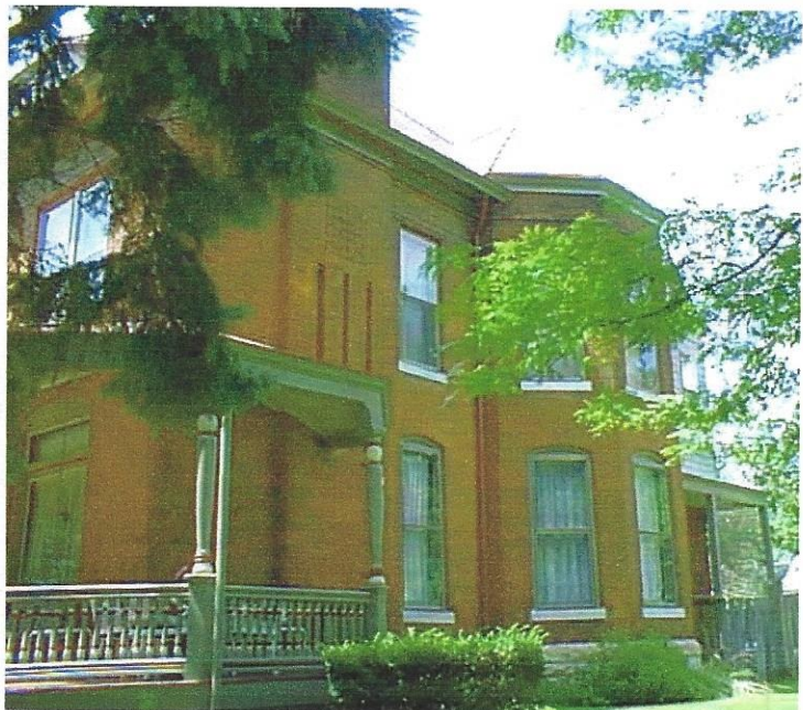
East side - chimney, turret, brickwork
