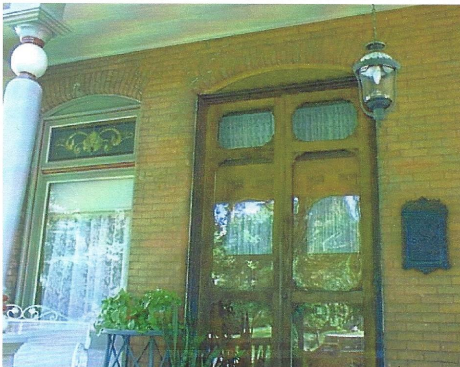
Entry detail - double door entry and transom windows, flat segmented arch brick lintels
