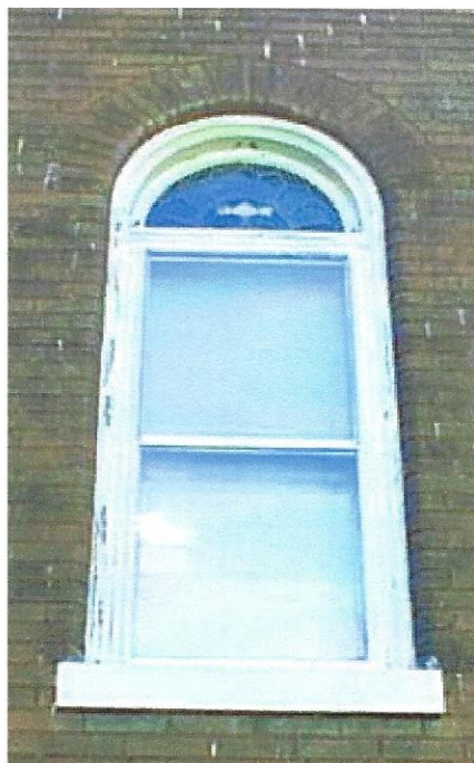
Arched window detail – relieving arch lintel, stained glass
