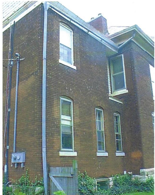
Rear addition , west side - middle chimney, brick relieving arch lintels, frieze, four over four panes
