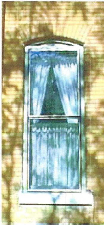
Window detail - flat segmented brick arch lintel, one over one sashes, stone sills
