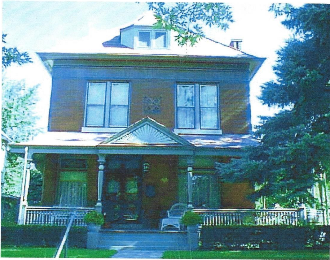
South facade - front porch, carved pediment detail, double door entry
