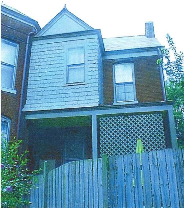
East side of rear addition showing shingled room
