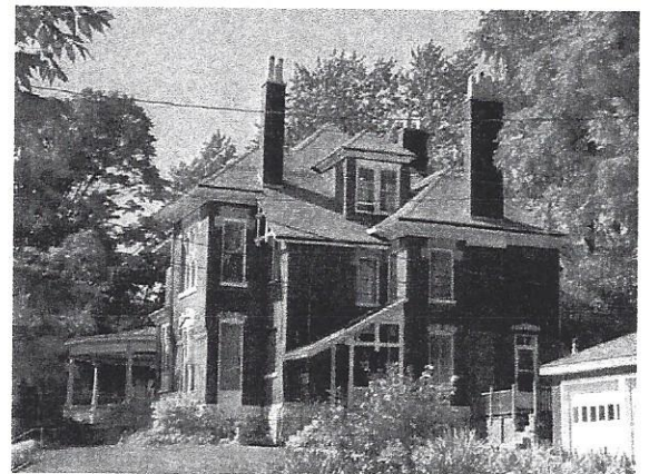
View from northeast showing roof massing and chimney placement.
