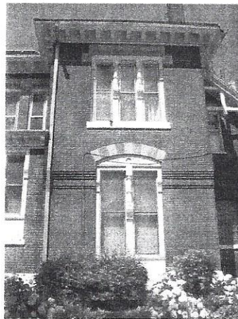
East bay. Preserve stone window hoods as well as eave brackets and Eastlake details around windows.
