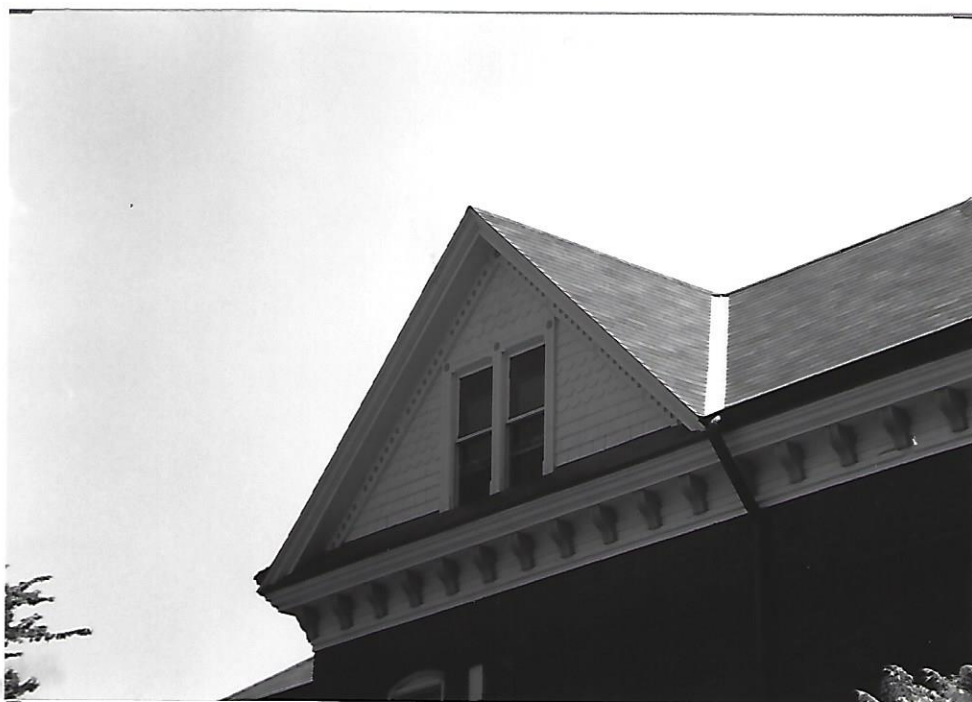
Detail of the North facade gable with wood shingles & decorative wood carving
