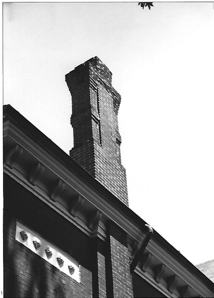
Detail of the chimney on the South facade with decorative brickwork
