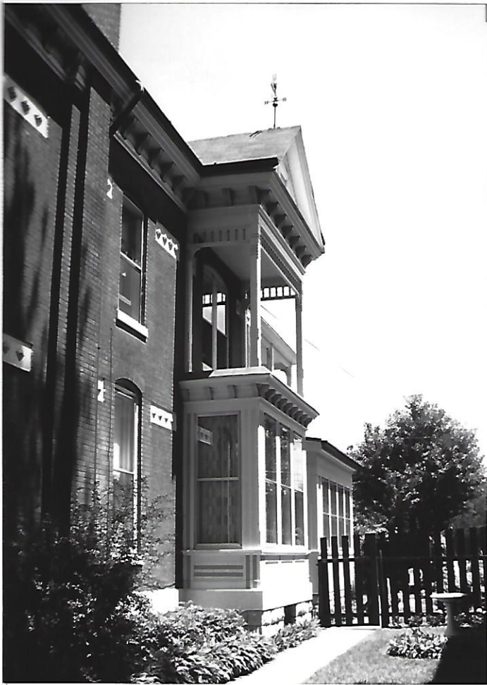
South Facade-Shows the rectangular bay with the two-story porch above with a gable roof
