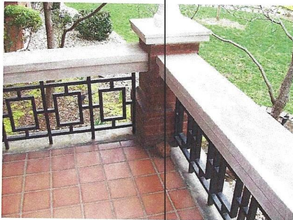
C2. Balustrade with cast iron panels and covered by broad limestone caps.
