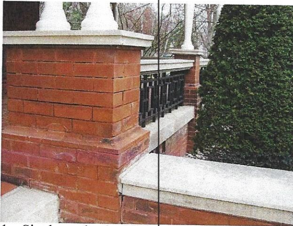
1a. Single- and paired Queen Anne columns resting on limestone-capped brick plinths with coved brick ledges.
