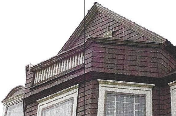
2c. Each porch has a balustrade with wooden square balusters.
