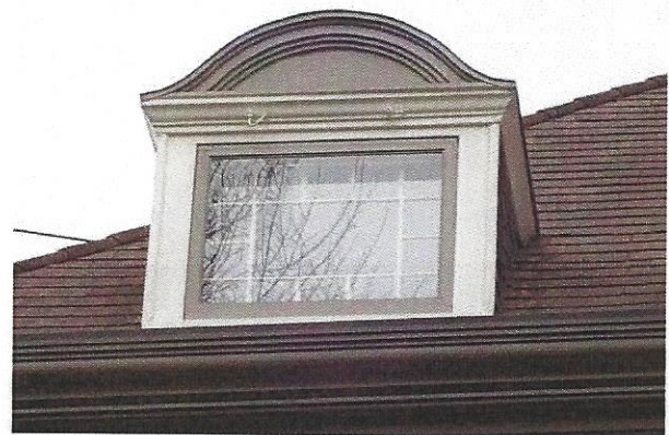
B3. Attic dormers with arched roofs—one facing north, and one facing south.
