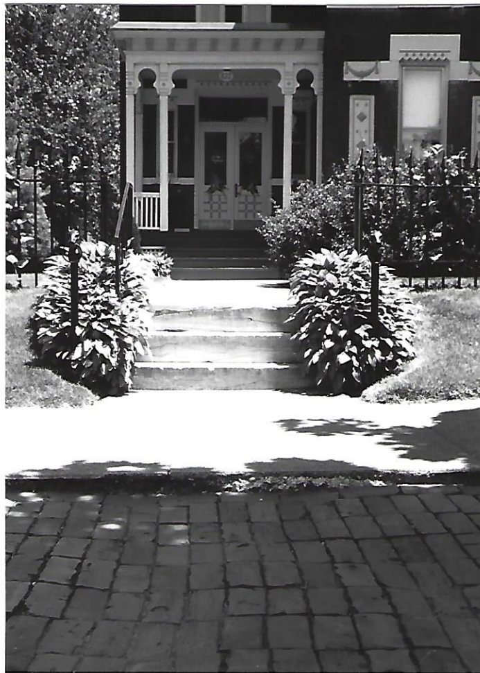
Detail of the stone steps and the brick walk between the city sidewalk and the street
