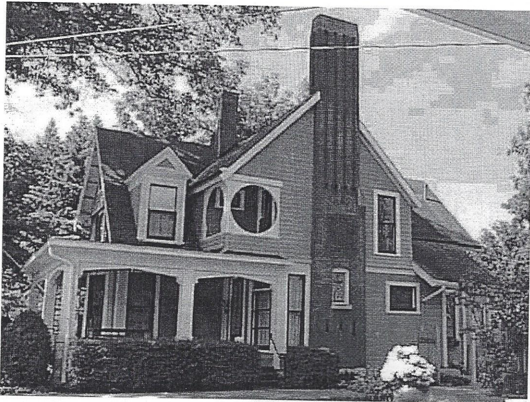
North side - decorative chimney, shingled gable, one over one double hung windows, porches
