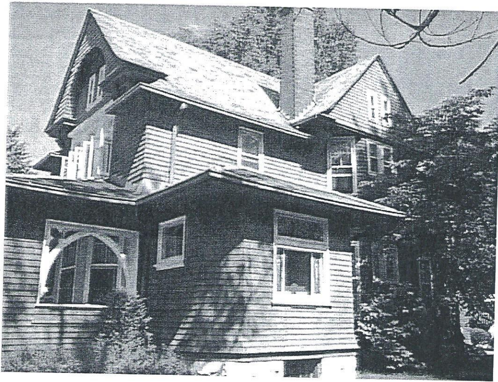
East facade - addition in front, bay window with gable top and paired windows, inset chimney
