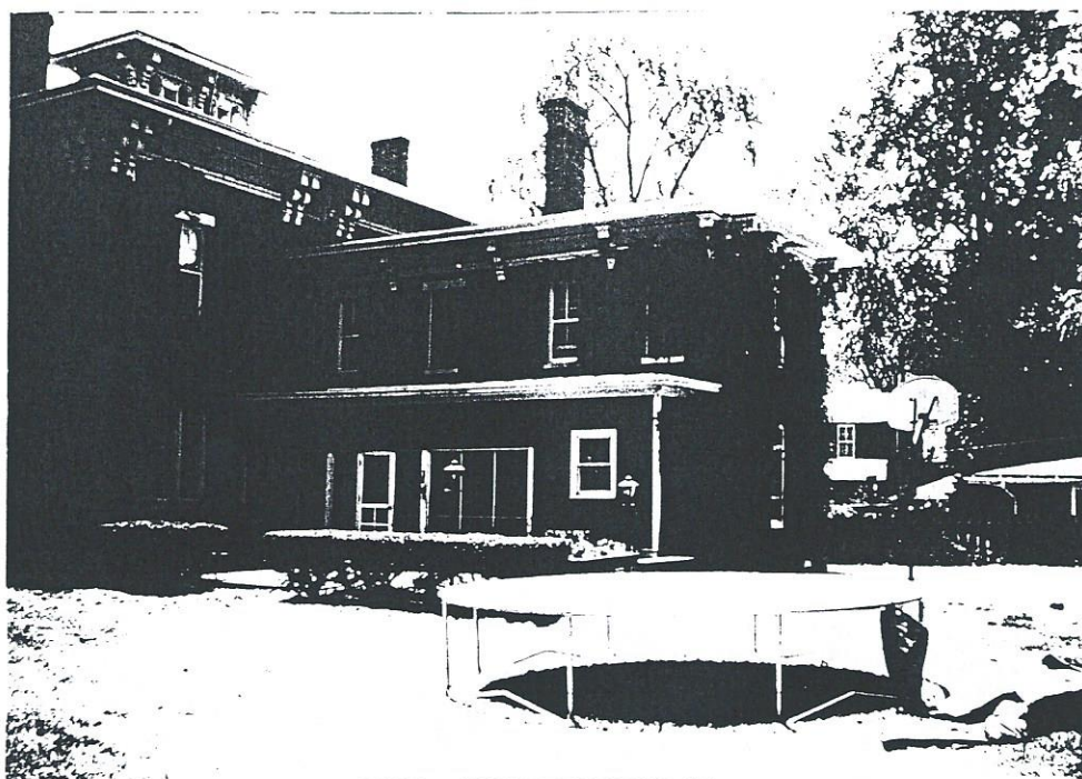
East Facade-Shows two-story addition to the rear with its chimneys, brackets, and window placement; also shows the North facade of the main mass of the house with its brackets and window placement
