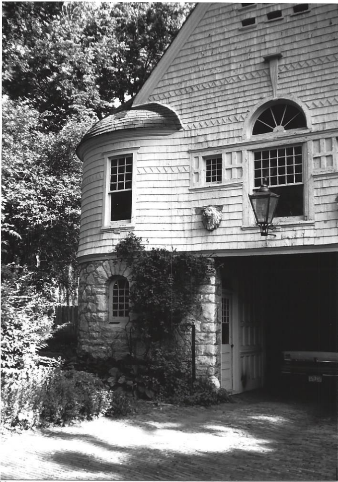
Detail of the carriage house tower from the South—Shows the stone first story and the wood shingle second story, and the dome roof, and the connection of the wall and tower
