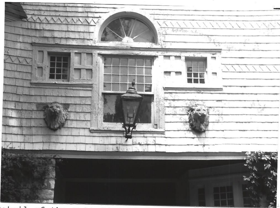
Detail of the Palladian window configuration on the South facade of the carriage house
