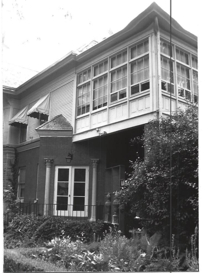
East facade-Shows the stone first story on the front and the brick first story on the rear with wood siding on the second story, also shows the second floor sleeping porch addition and the garden entry that protrudes at an angle
