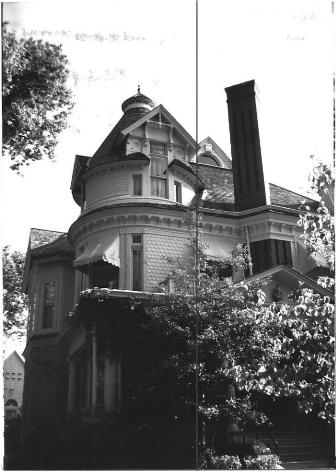
Detail of the tower on the Southwest corner with conical roof, conical cap and finial, windows and decorative dormer with turned wood truss, brackets, and carving
