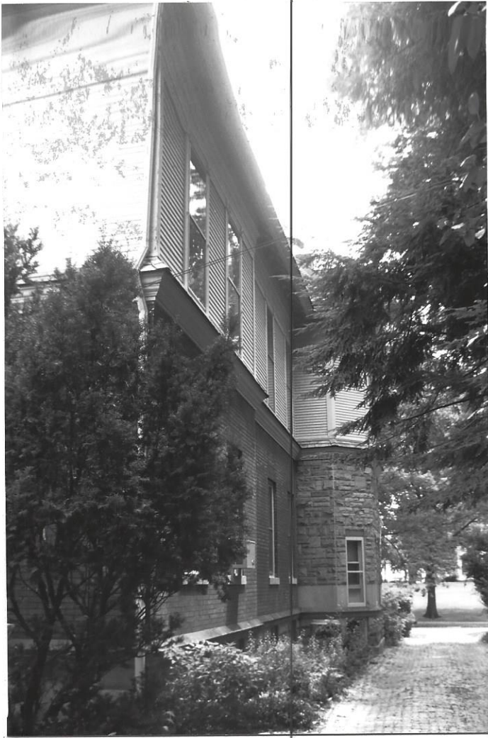
West facade-Shows the stone first story from the front and the brick first story on the rear with wood siding on the second story, also shows the placement of windows and the brick drive on the West edge of the property
