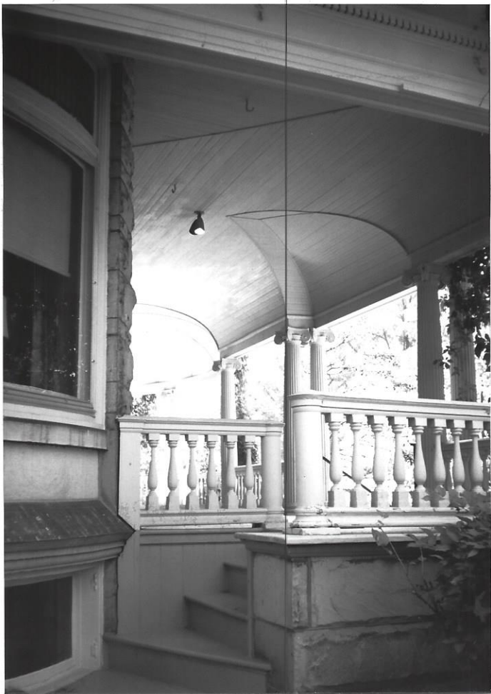
Detail of the wrap-around porch-Shows the wood vaulted ceiling, Ionic columns, wood rail and turned wood balustrade, also shows the wood steps leading from the drive to the West
