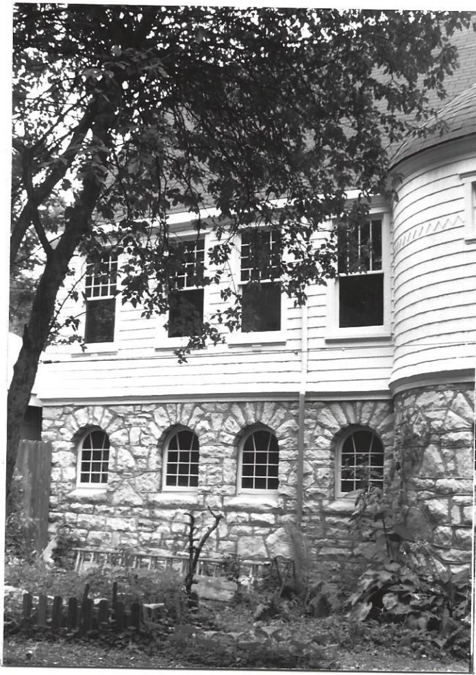
West facade of the carriage house-Shows the stone first story and the wood shingle second story, the placement of window openings and the connection of the wall and tower
