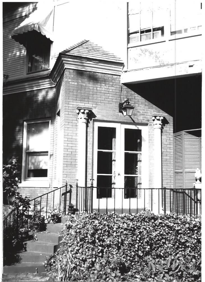
Detail of the garden entry on the East facade that protrudes at an angle; the double doorway is flanked by Corinthian columns
