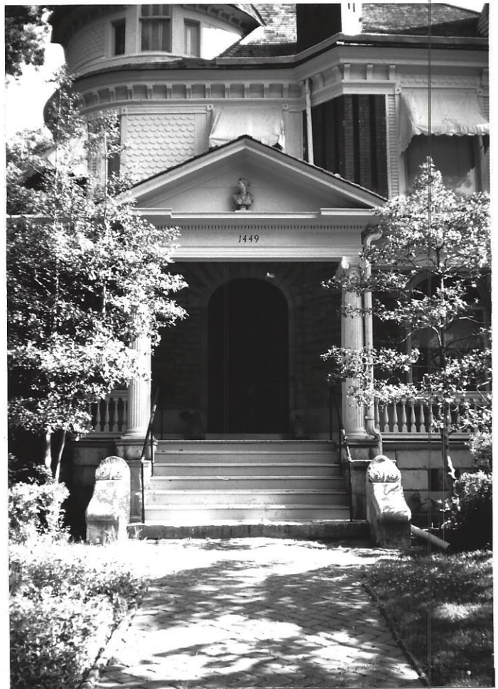
Detail of the pediment above the front steps to the porch-Shows the wood front steps and the semi-circular arch door opening beyond
