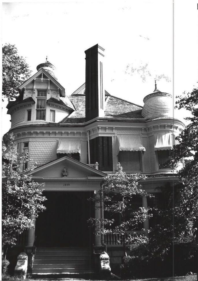
South facade-Shows the chimney with decorative brickwork, also shows the tower, turret, and porch
