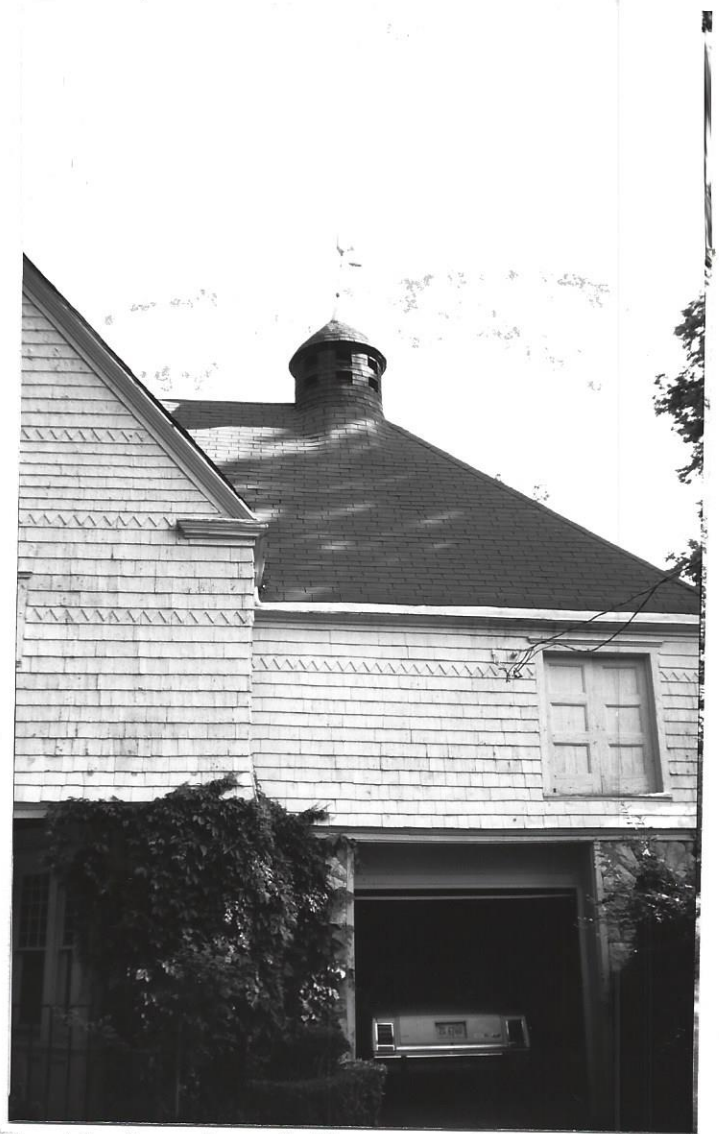
South facade of the carriage house- Shows the stone first story, the wood shingle second story, the hip roof, and dovecote
