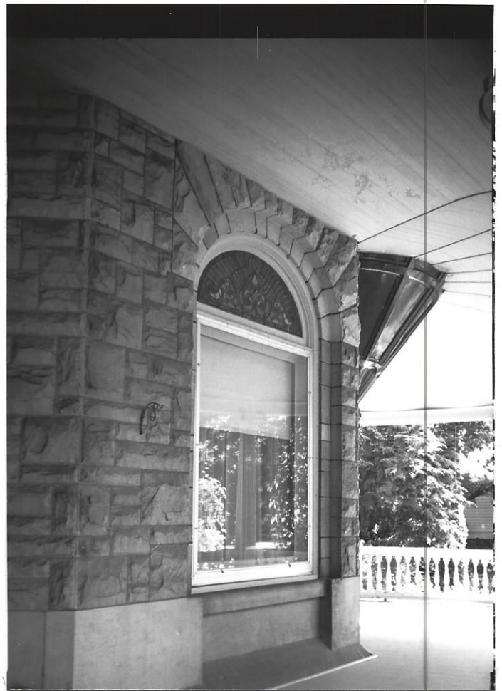
Detail of a first story window on the South facade with semi-circular stone arch opening, leaded glass toplight and plate glass window below
