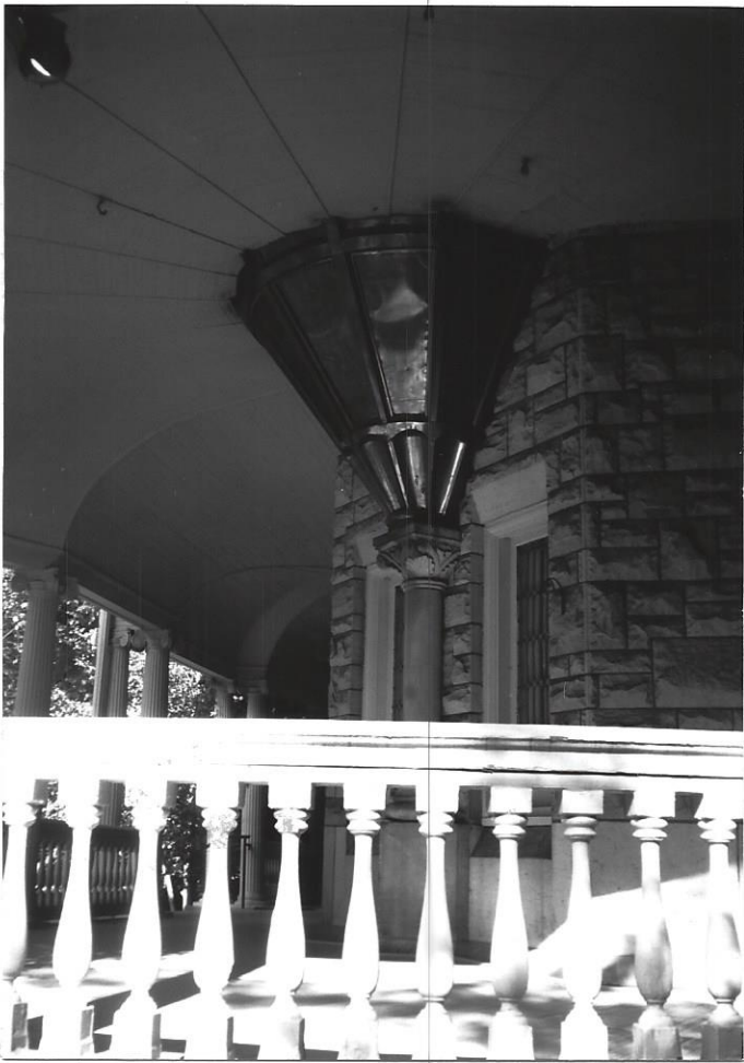
Detail of the porch-Shows the Composite column with copper molding above, the vaulted ceiling the the wood rail and turned wood balusters
