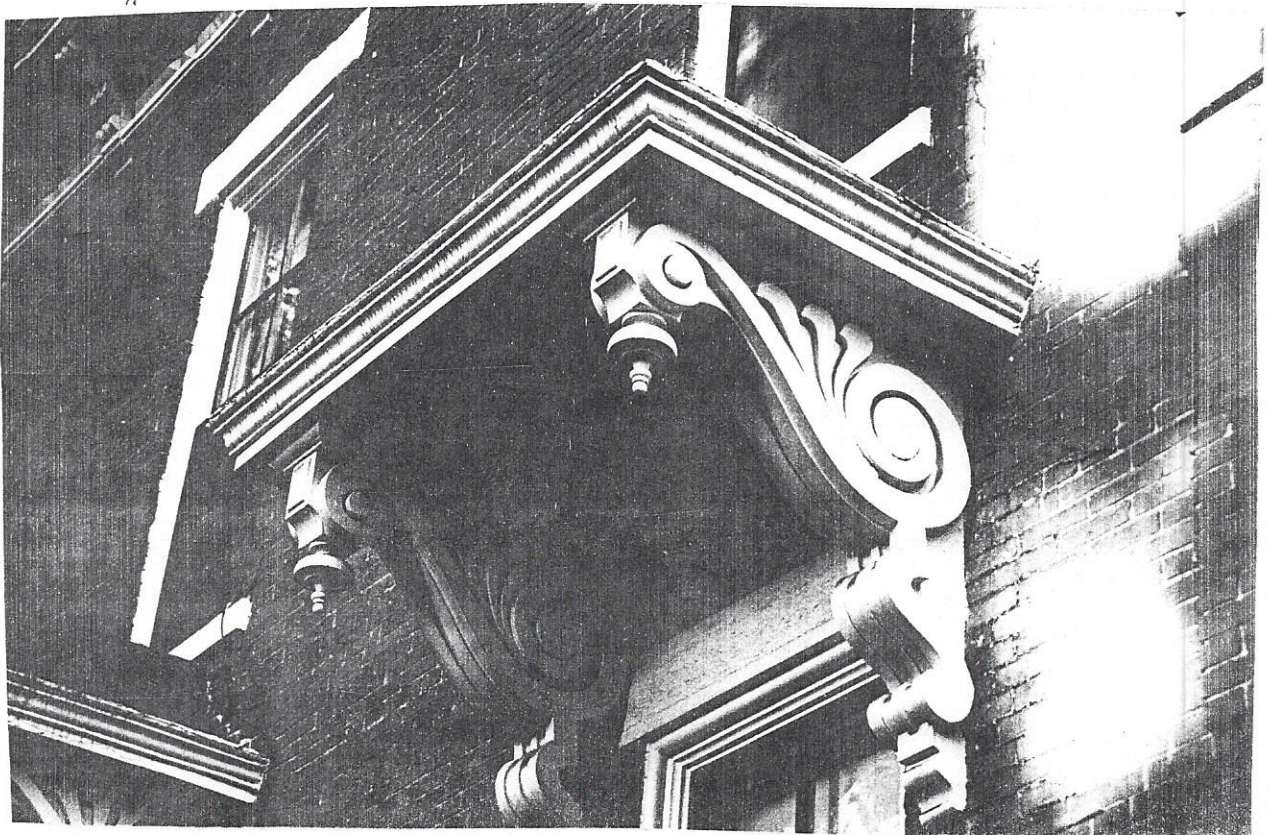
EAST SIDE BALCONY DETAIL
